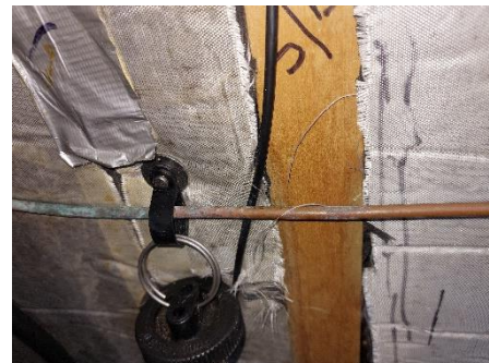
Gas pipework not supported and with corrosion.
