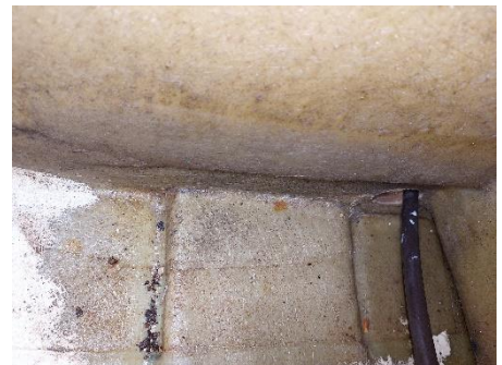
Re tab torn laminate as noted.
