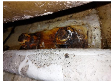
Obvious corrosion to Stbd fastenings.
